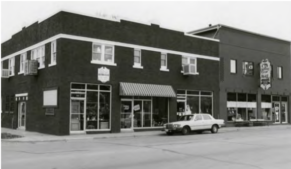
Cazzell Building #2, 2801 S Georgia St., 1993
