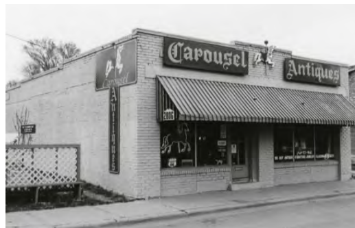
Cazzell Building #1, 2806 S Georgia St., 1993
