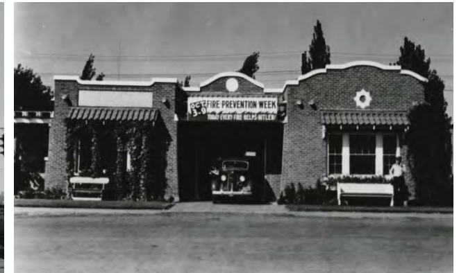
San Jacinto Fire Station, 610 S Georgia St., c. 1940
