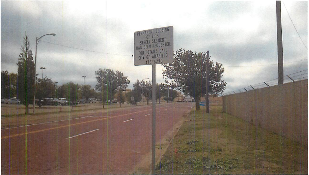
Photos taken days later when notice signs were posted, looking down SE 7 th Ave in front of City Hall.
