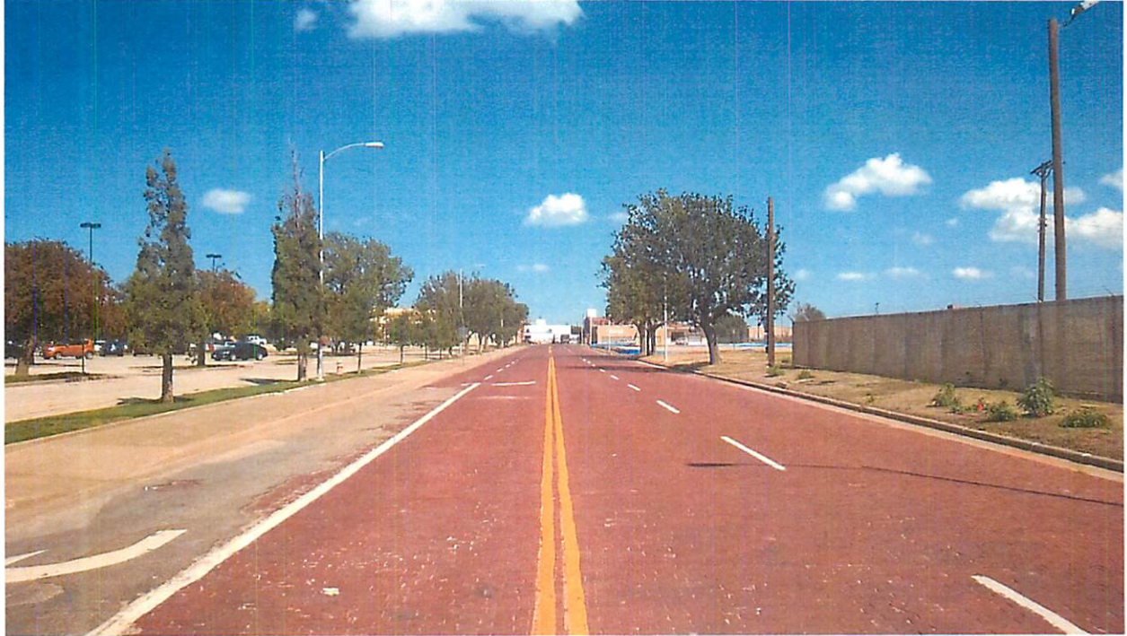
Looking east down SE 7 th Avenue in front of City Hall.
