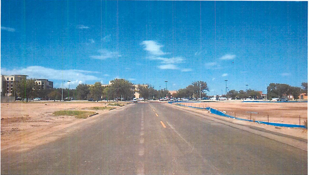
Looking north up S Lincoln Street (80' ROW) towards City Hall.
