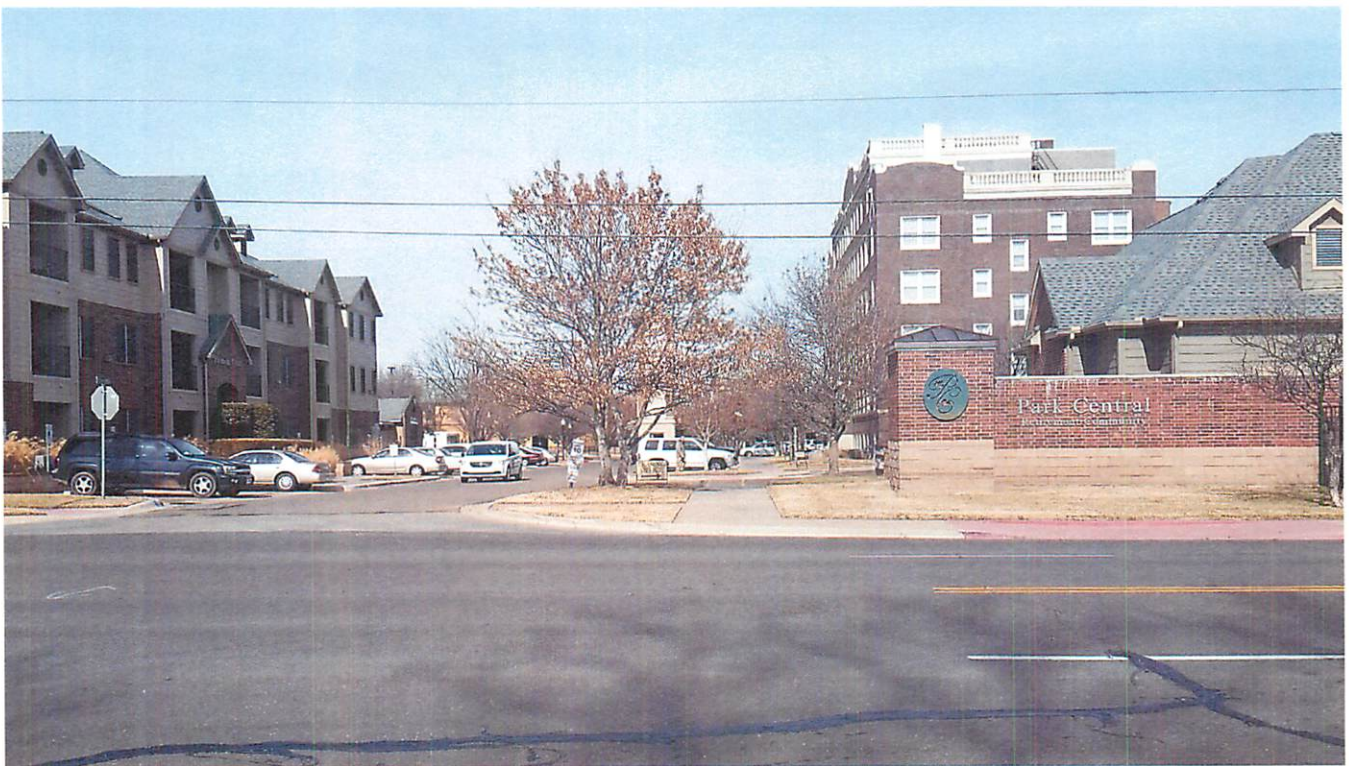
Looking north from S Van Buren St. & SW 15 th Ave. at retirement community campus.
