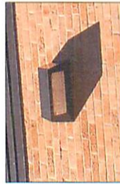
A TYPICAL EXTERIOR BUILDING LIGHT
