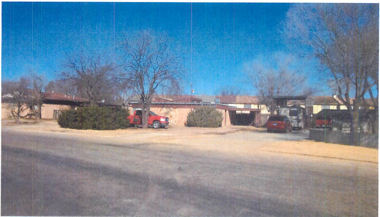
Looking north across the street (Mays Avenue) from the property for consideration.
