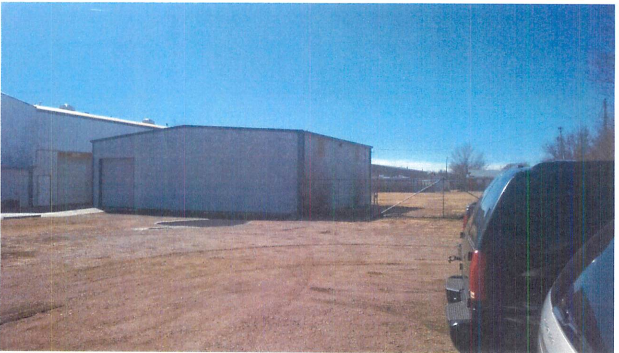
Looking southeast next door (Subject property is to the right), this is zoned Light Industrial (I-1).
