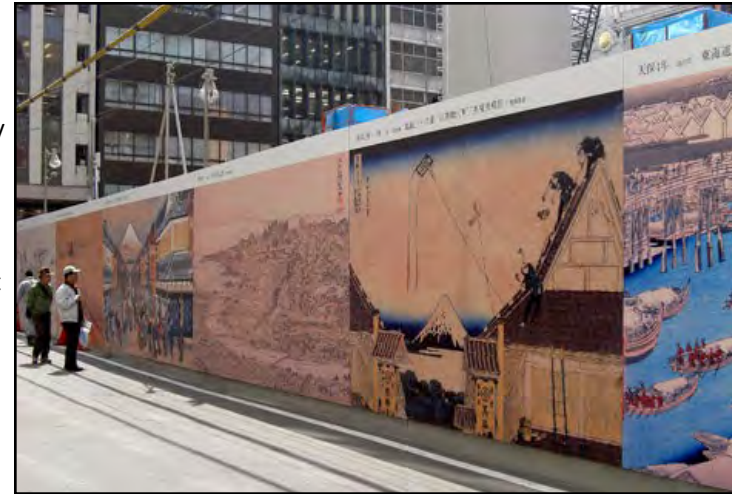
Temporary construction fences can add interest to downtown by utilizing renderings of the project or artistic images.
