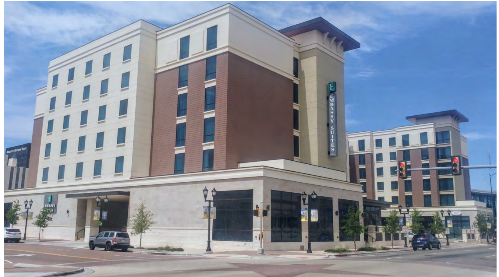
Convention hotel opened in September 2017 across the street from the Amarillo Civic Center
