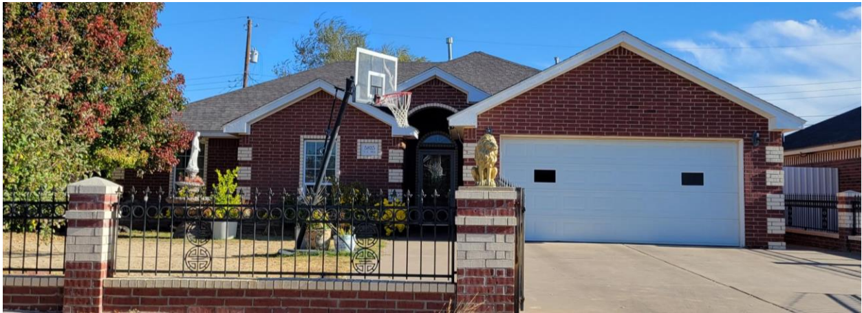
Figure 86: Existing Single family Properties
