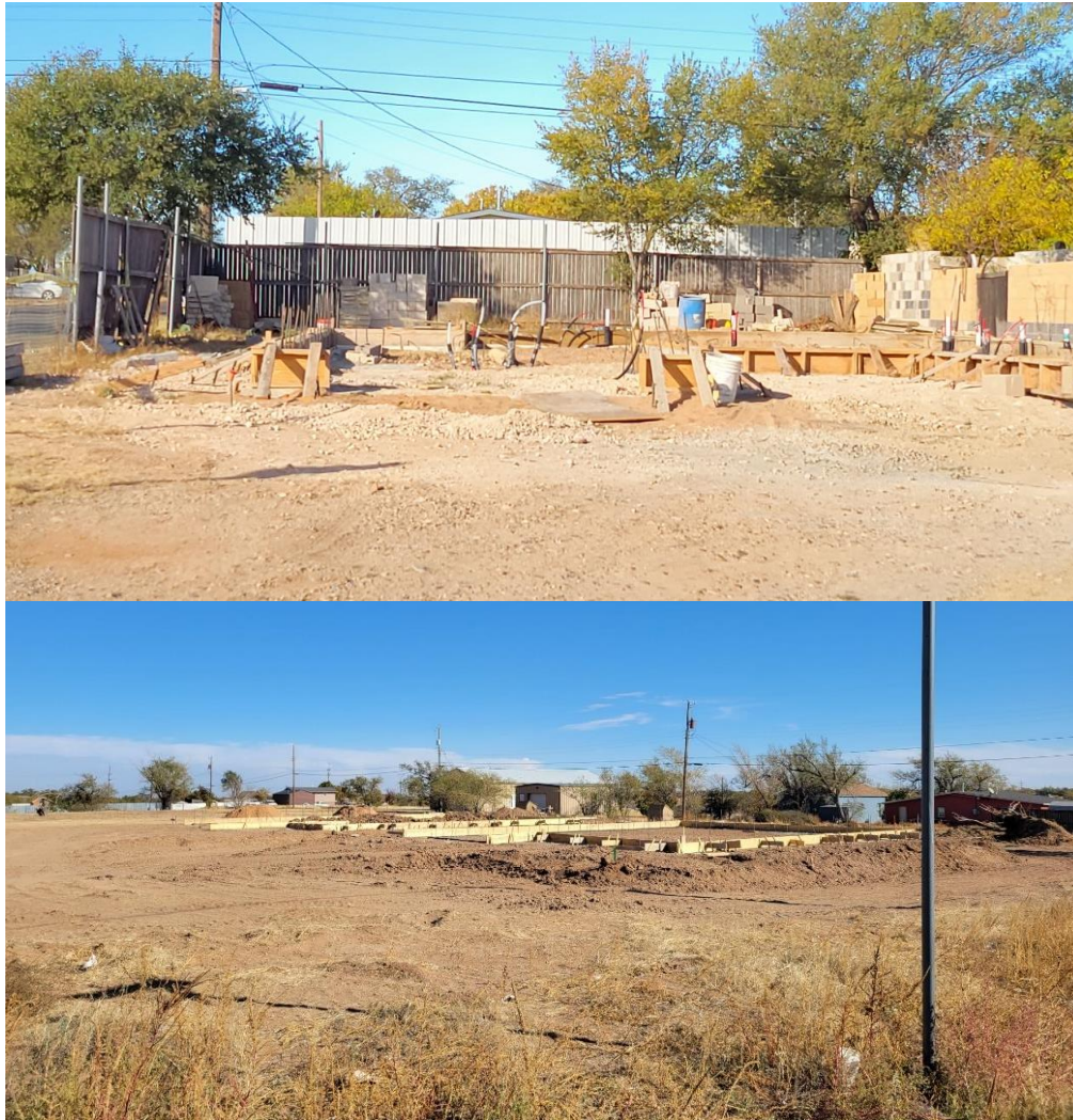
Figure 87: New Single family Infill Construction
