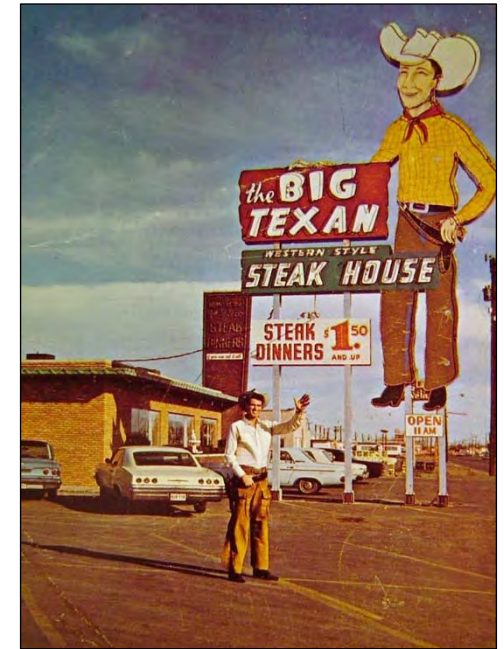
Original Big Texan Building, 1962
