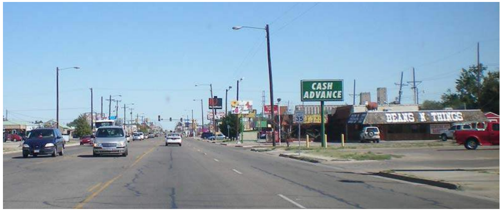
Older segments of Amarillo Boulevard illustrate the lack of access management controls in earlier arterial construction, even on roadways designated as U.S. and/or State highways (Business 40 in this case). The proliferation of driveways along a major thoroughfare, together with a continuous center left turn lane, not only detracts from smooth traffic flow, but each driveway (along with intersecting side streets) creates a potential conflict point between entering and exiting vehicles and pedestrians and bicyclists moving along the arterial.
