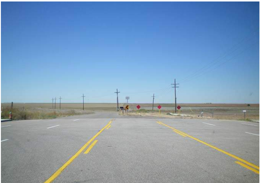
This view at the current western terminus of SW 45 th Avenue highlights the importance of orderly extension of the thoroughfare network, in conjunction with new growth and land development, such as may occur to the west of Soncy Road in coming years.
