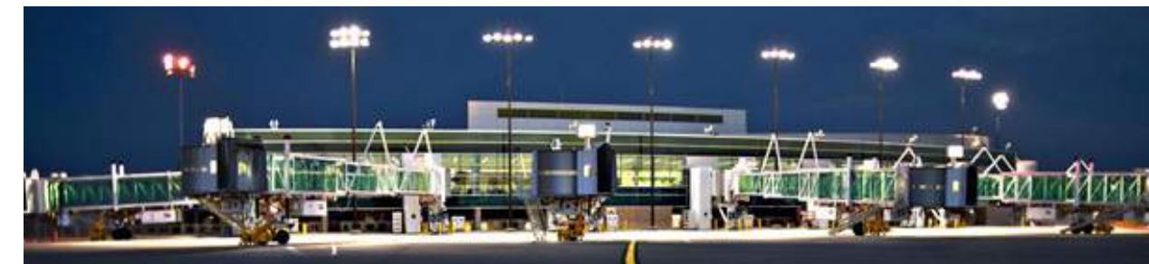
Figure 6-7. Rick Husband Amarillo International Airport
