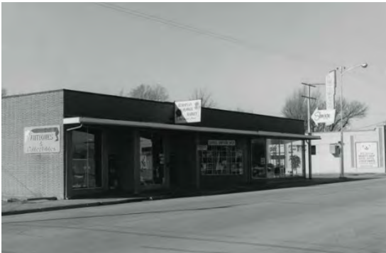
Gussler Products Building, 2917-25 SW 6 th Ave., 1993
