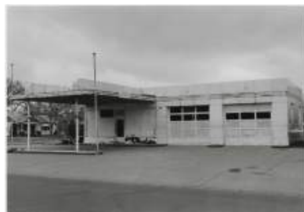
Taylor's Texaco Station, 3512 West Sixth, 1993
