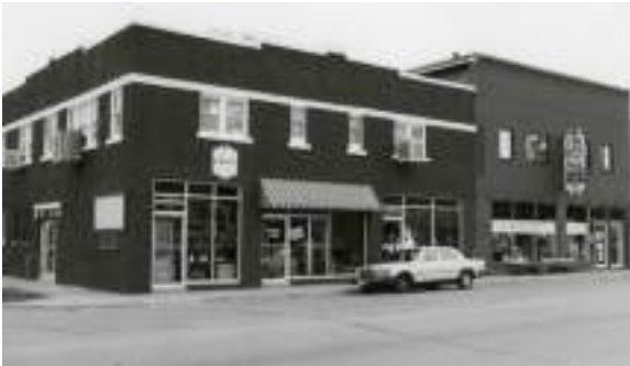
Cazzell Building #2, 2801 South Georgia, 1993
