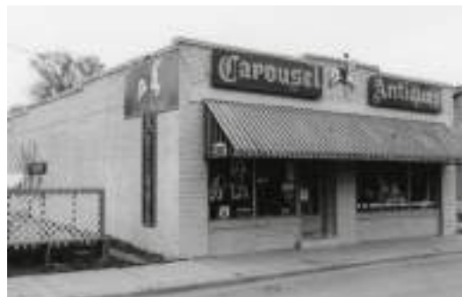
Cazzell Building #1, 2806 South Georgia, 1993
