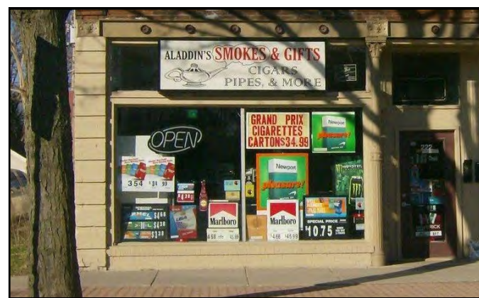
An example of signage clutter
