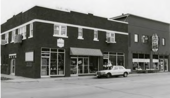
Cazzell Building #2, 2801 South Georgia, 1993
