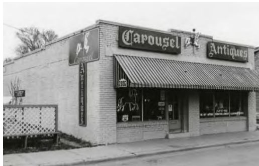
Cazzell Building #1, 2806 South Georgia, 1993
