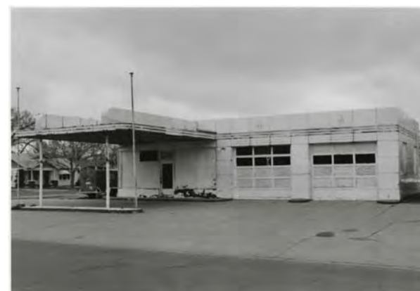
Taylor's Texaco Station, 3512 West Sixth, 1993
