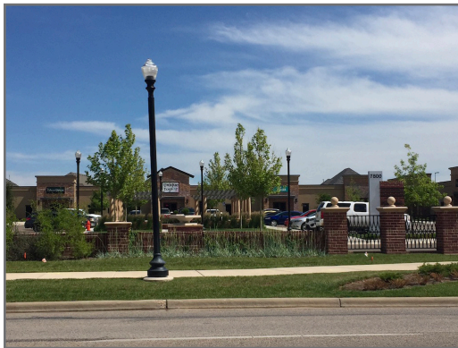
Although landscaping adds to upfront development costs, it enhances a site's appearance and can contribute to increased property values.
