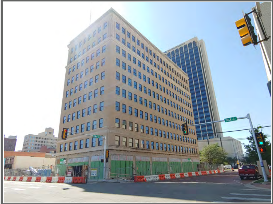
Barfield Building (During Renovation)
