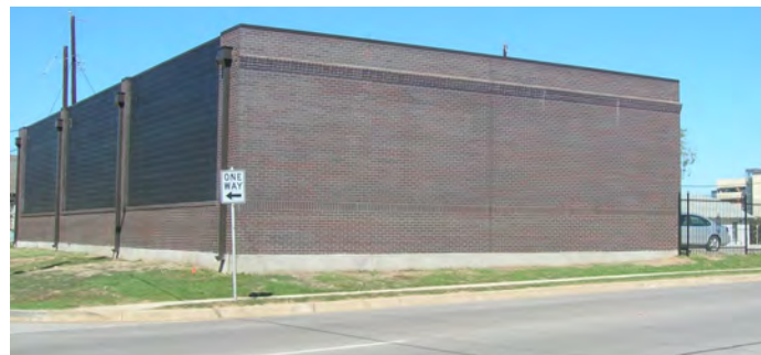
Facades facing the street and/or pedestrian walkway without transparency and architectural articulation are not allowed
