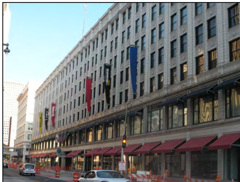
A comprehensive building signage plan helps ensure continuity in the façade.
