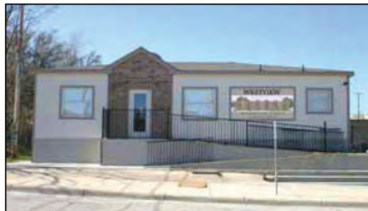
Temporary construction trailer
