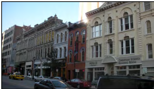
Buildings that are located at or near the property line and have varying architectural articulation create interest for downtown users.
