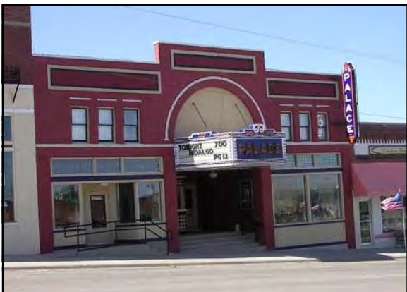
Marquee signs are typically installed on theaters, cinemas and performing art facilities.
