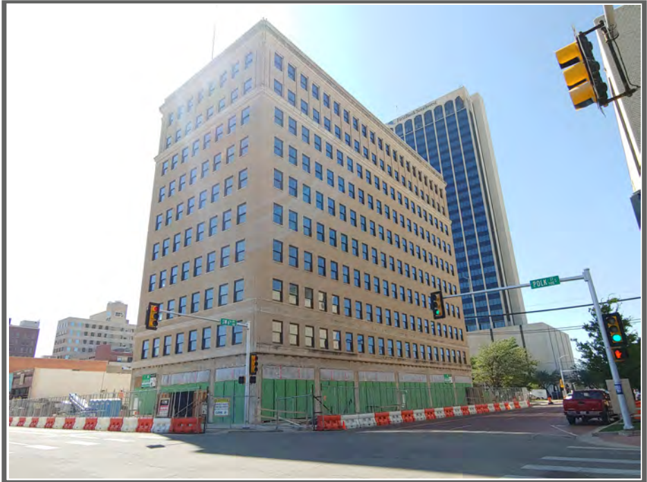
Barfield Building (During Renovation)
