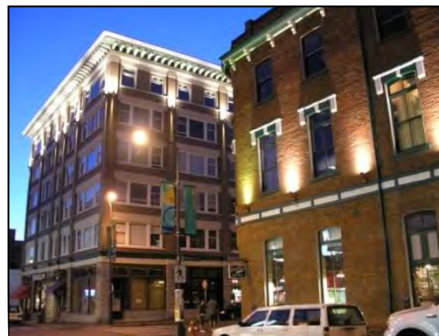
Exterior lighting can accent architectural features and is encouraged.
