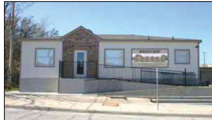
Temporary construction trailer
