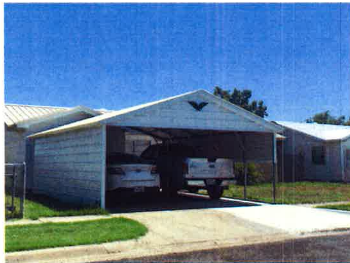
Neighboring carport to the north with no specific use permit:
