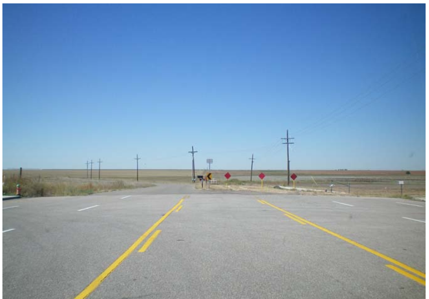
This view at the current western terminus of SW 45 th Avenue highlights the importance of orderly extension of the thoroughfare network, in conjunction with new growth and land development, such as may occur to the west of Soncy Road in coming years.
