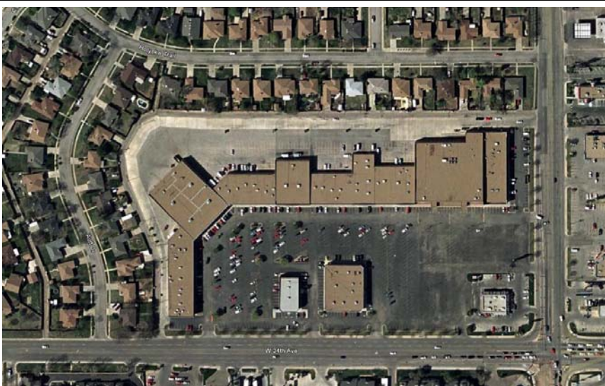
In the classic Auto Urban pattern, retail centers (such as this example at SW 34 th and Coulter) often have their principal buildings pushed to the rear of the site to focus parking and pad site uses toward the frontage. This can create compatibility issues with adjacent homes, especially since this often places delivery, loading, and trash collection activity nearest to the immediately abutting residential uses.
