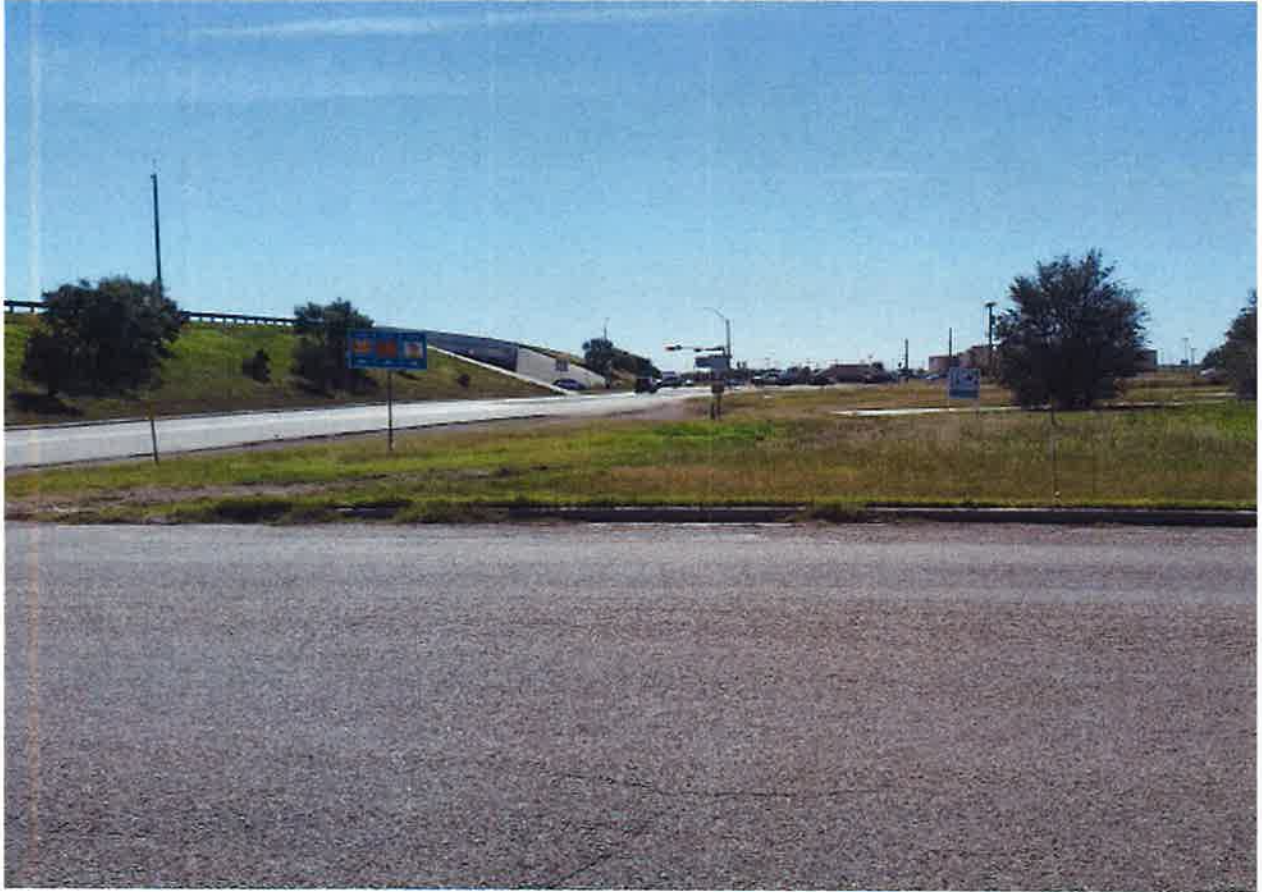
Looking south from IH27 & Thunder Rd at major intersection.
