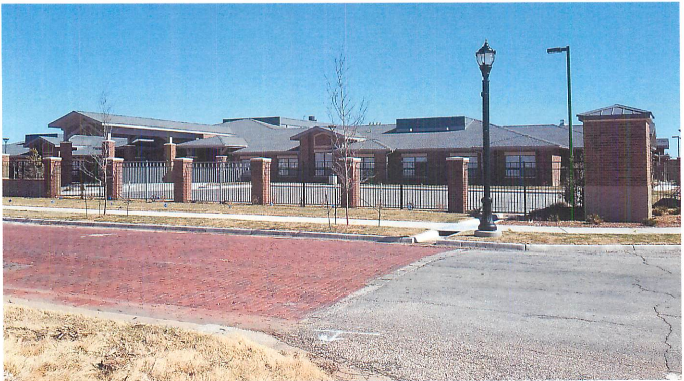
Looking northeast from S Van Buren St. & SW 16 th Ave. at Park Central Memorial.
