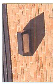
A TYPICAL EXTERIOR BUILDING LIGHT
