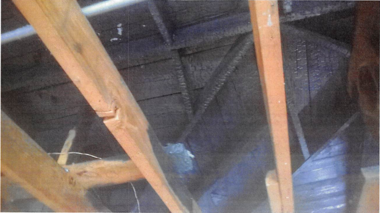
Interior Fire Damage above the Kitchen:
