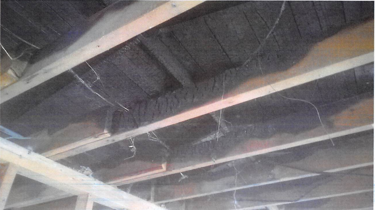
Interior Fire Damage above the Kitchen:
