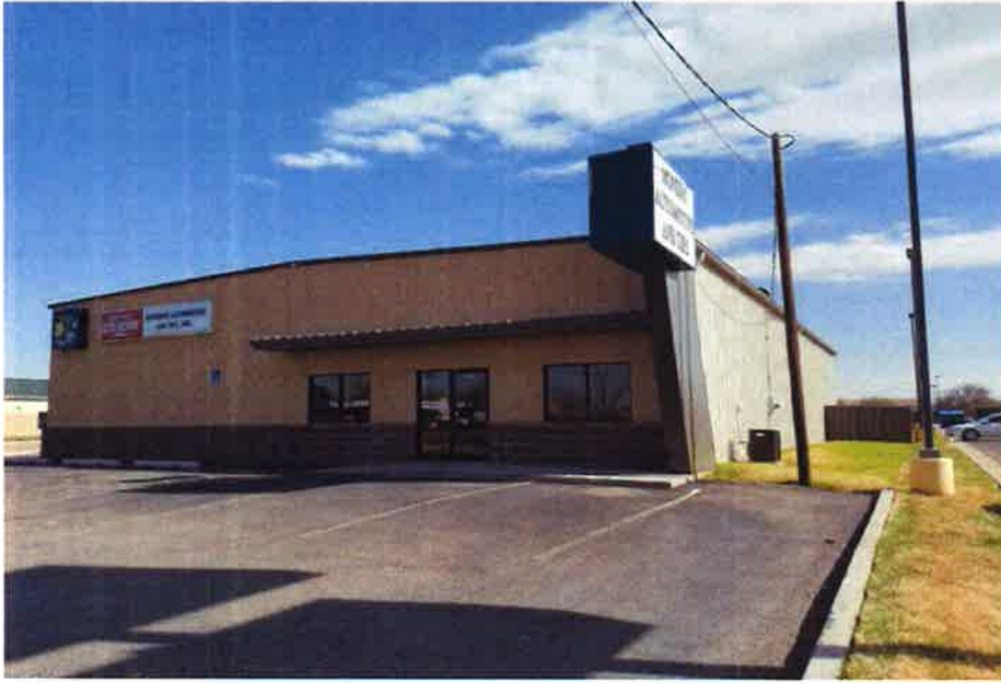
Existing Auto Repair building to be remodeled and an addition added .
