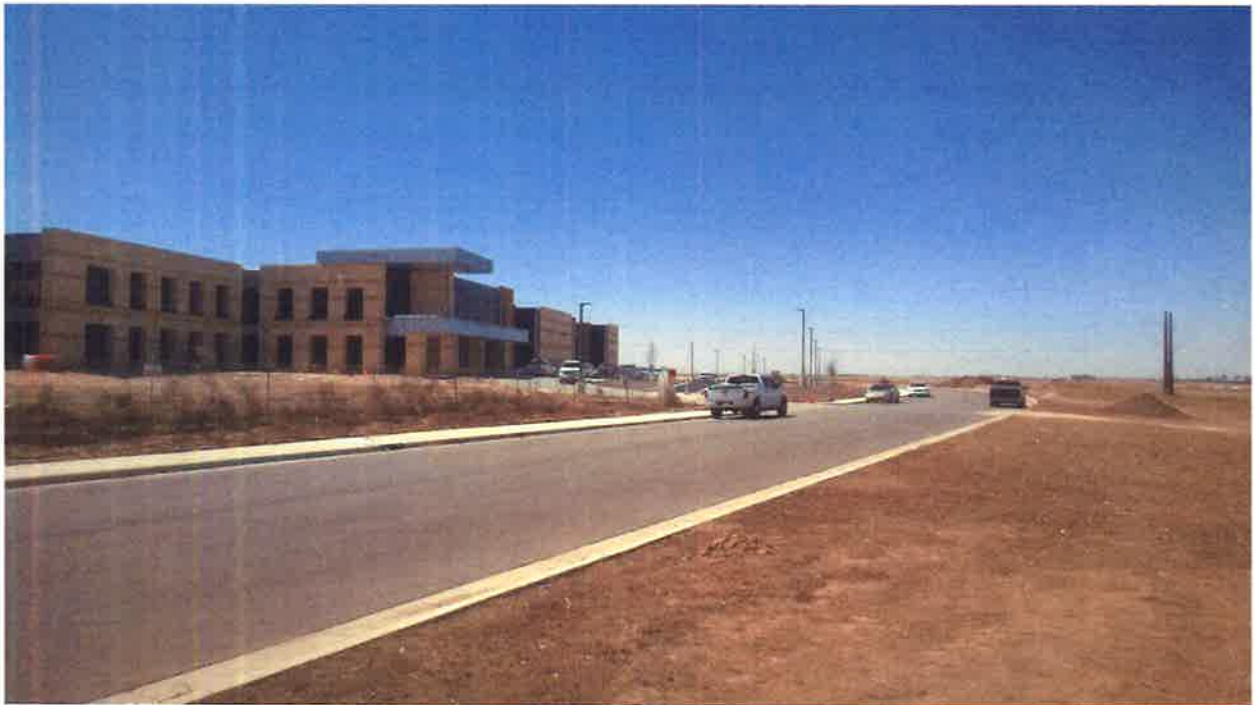
Looking west from Meadow Ridge Drive down the PUE for consideration (CISD Intermediate School)
