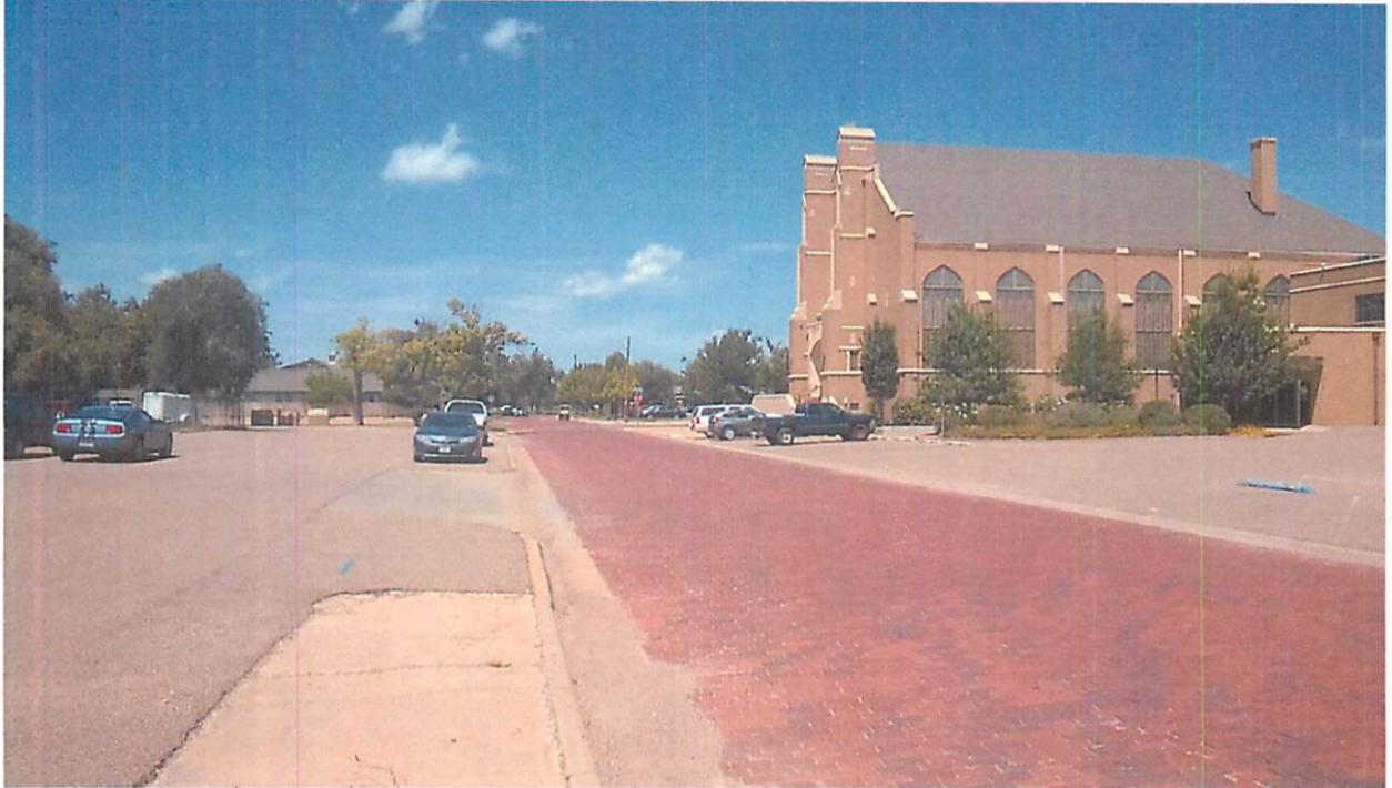
Looking northeast up S Monroe St, which is 80' wide of ROW. Bricks are to be recycled.
