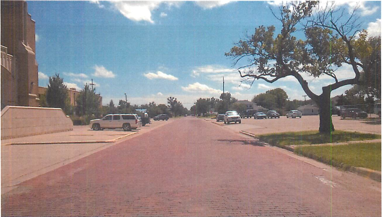
Looking south down S Monroe St, which is 80' wide of ROW. Bricks are to be recycled.
