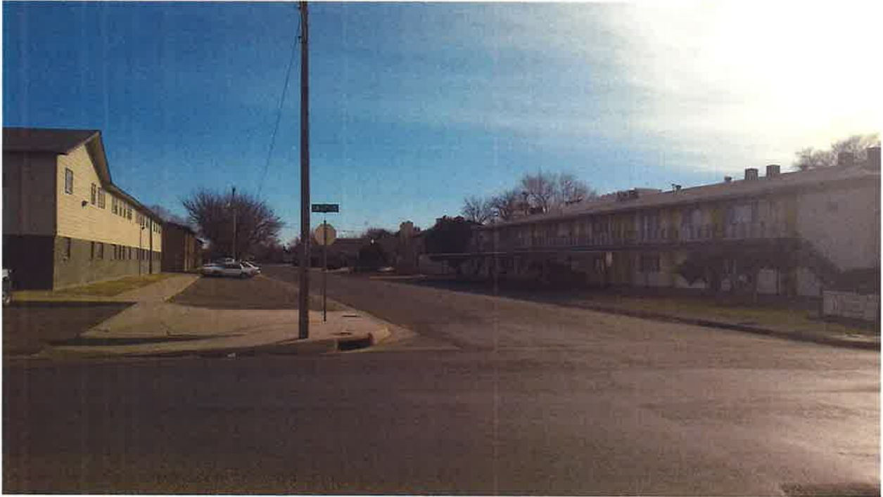
Looking south down Britain Drive from the proposed rezoning tract, MF-1 zoned apartments.
