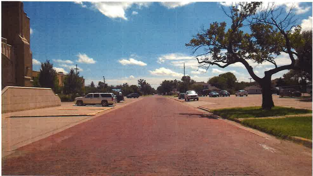
Looking south down S Monroe St, which is 80' wide of ROW. Bricks are to be recycled.
