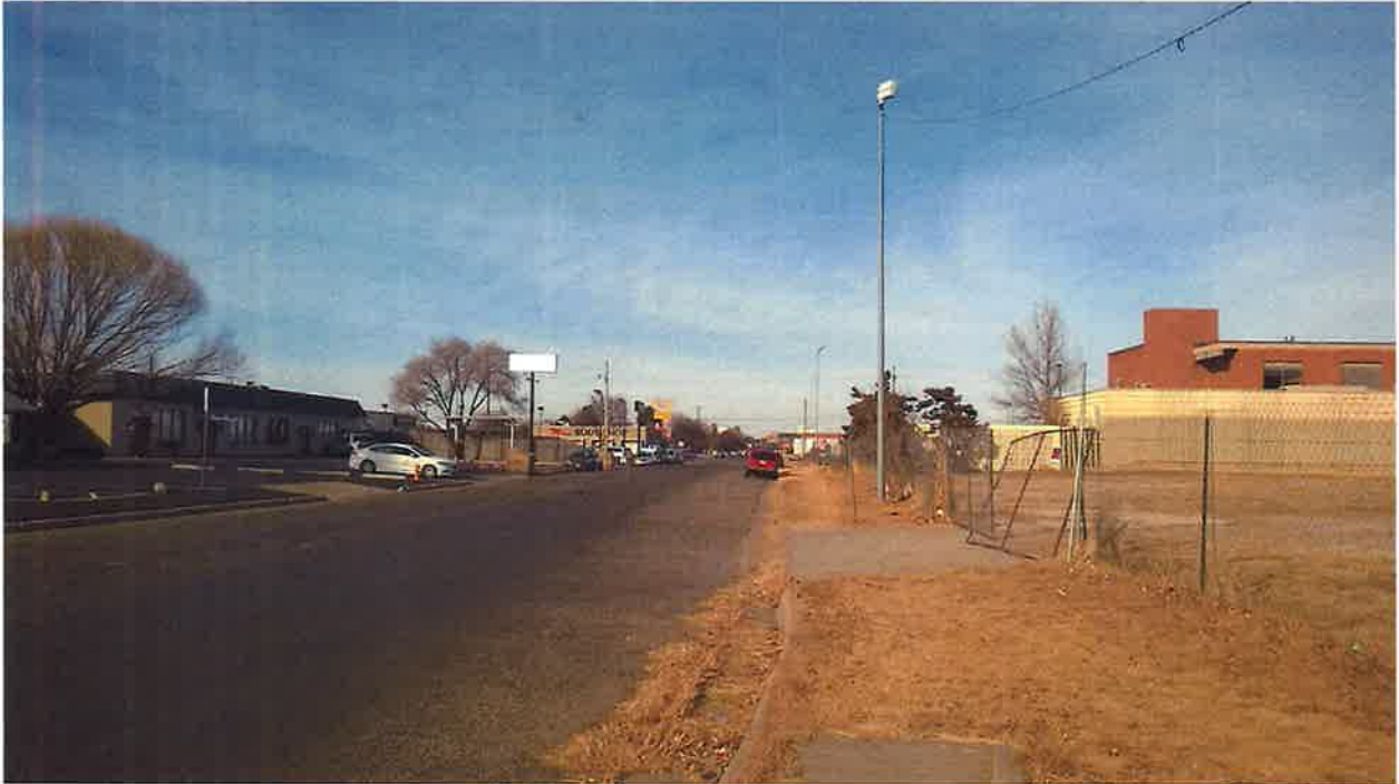
Looking north of Britain Drive from the SW corner of the proposed rezoning tract, GR and LC on the left and applicant's property on the right.
