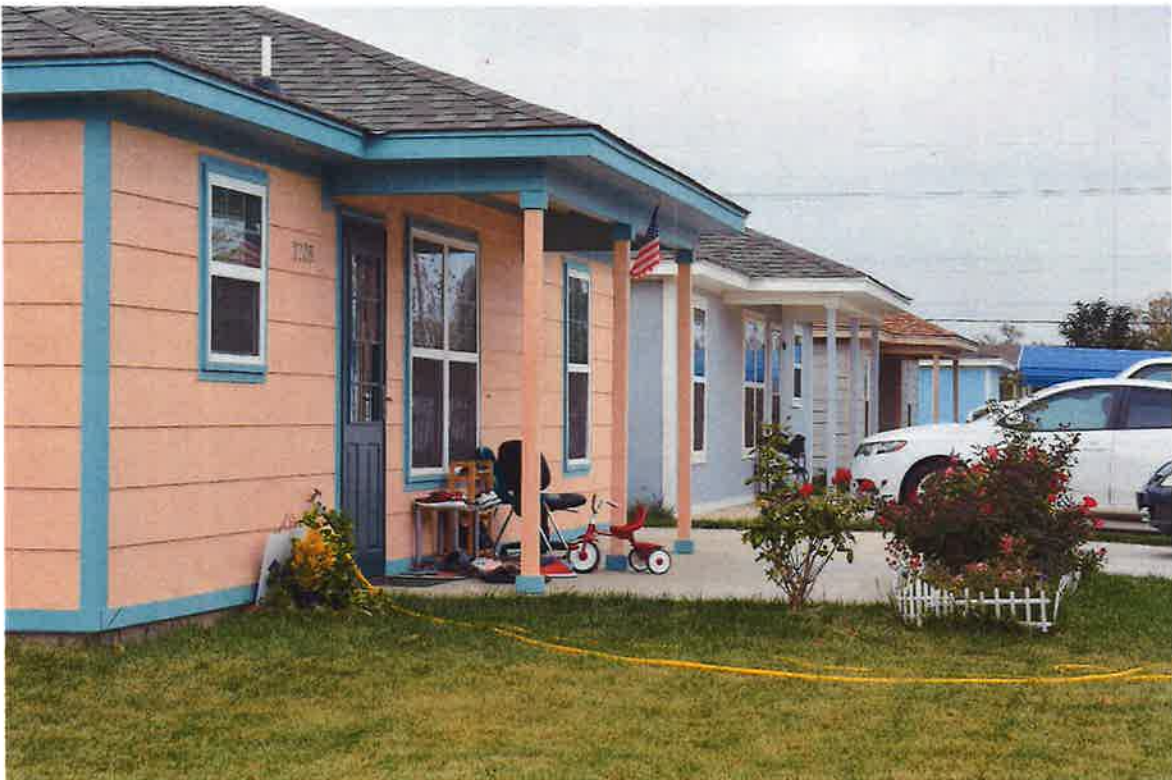
Glenwood Addition After
