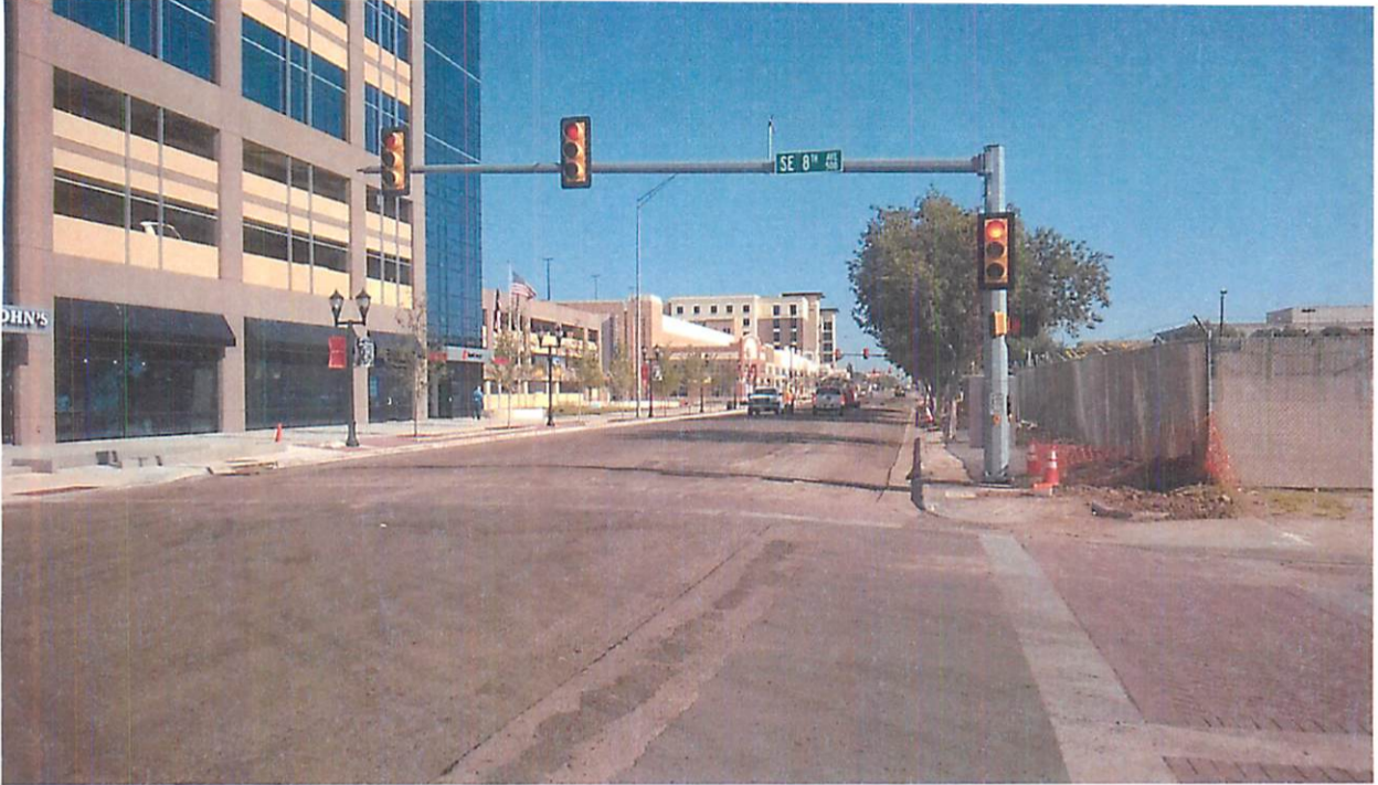
Looking north up S Buchanan Street, Xcel Energy building seen left and MPEV site seen right.
