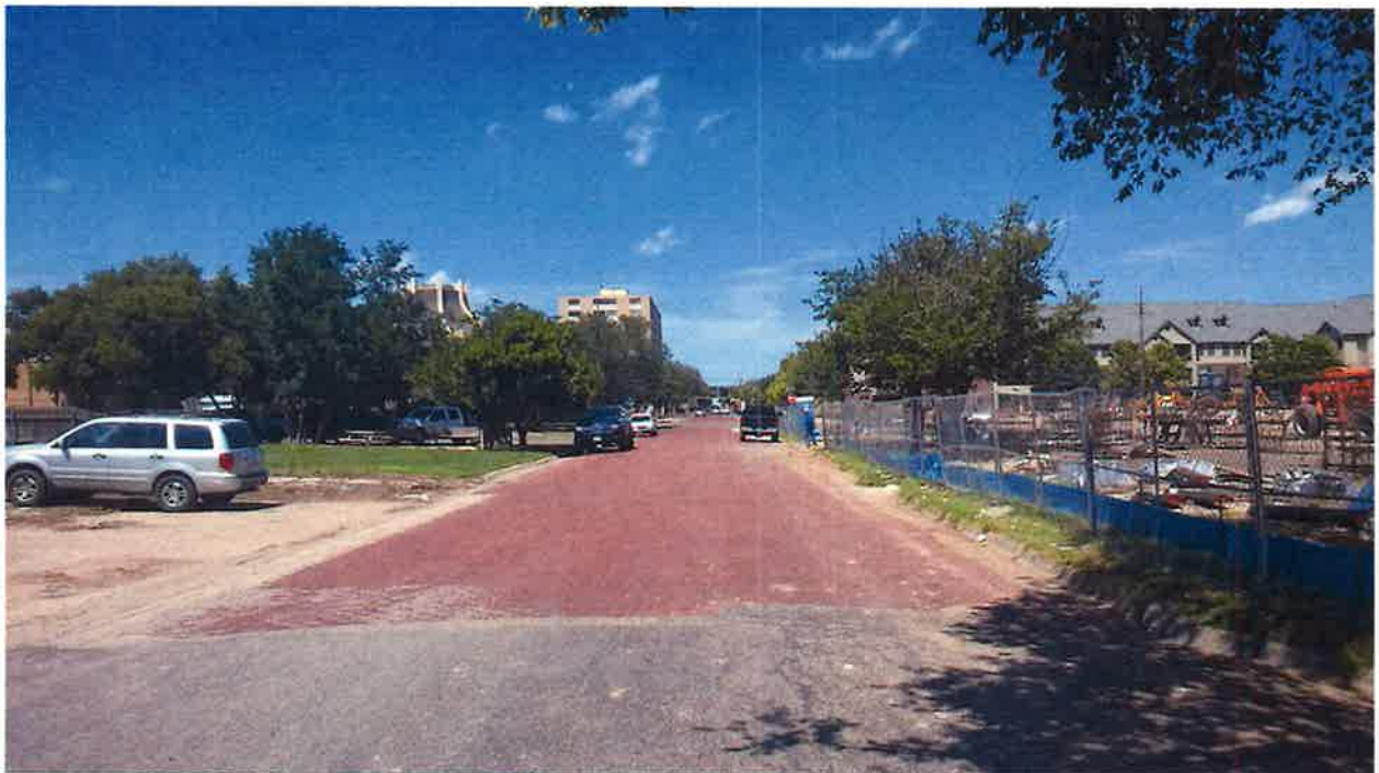
Looking north up S Jackson St from the intersection of SW 16 th Ave and S Jackson St. (BCS Campus on Right)
