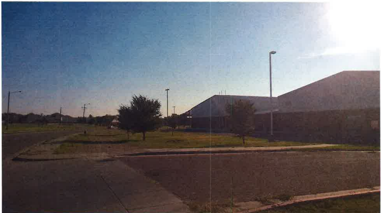
Looking northeast from SW 58 th Ave towards the existing netplex building that is under consideration.
