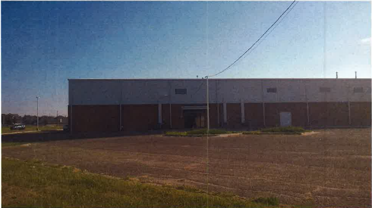
Looking northeast towards the existing netplex building that is under rezoning consideration.
